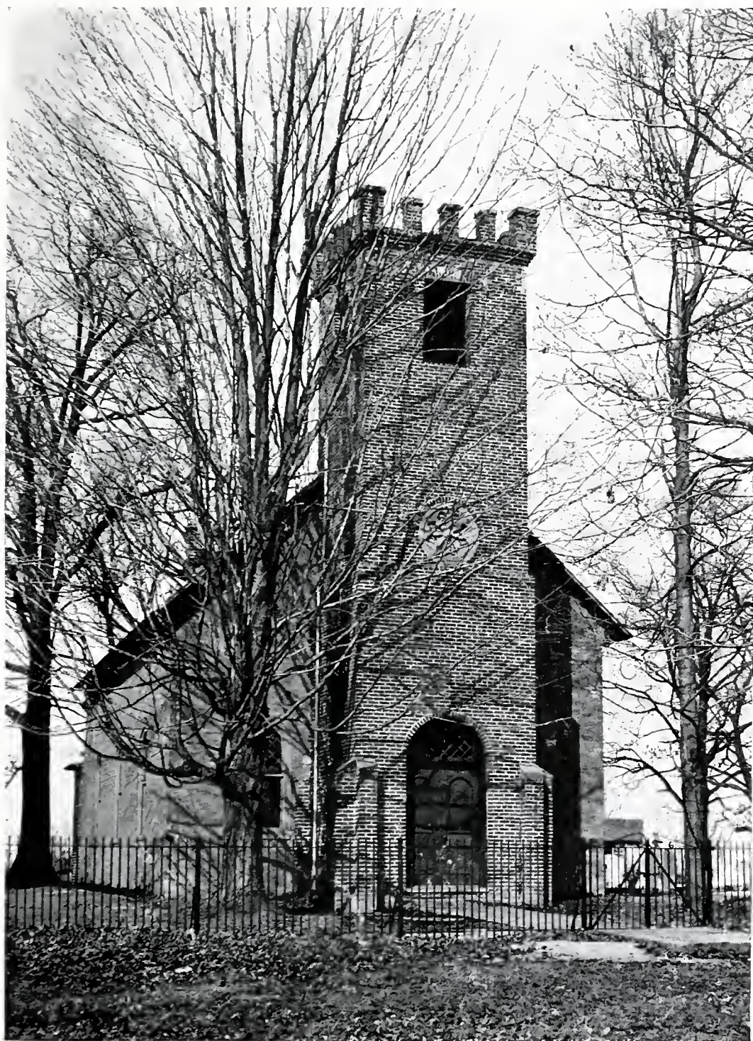
SHREWSBURY, BUILT 1832 LOCUST GROVE, KENT COUNTY
